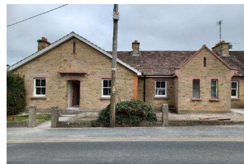
14 cottages being restored at St. Ita's, Portrane
